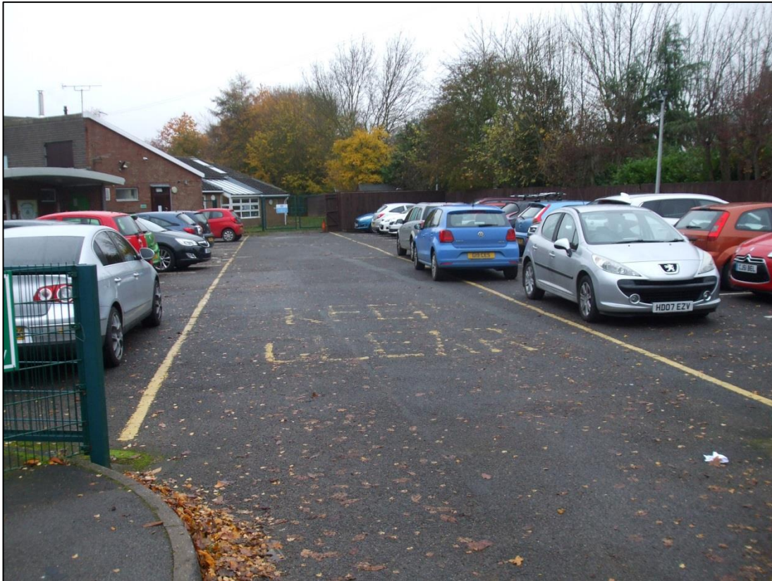
Existing Car Park
